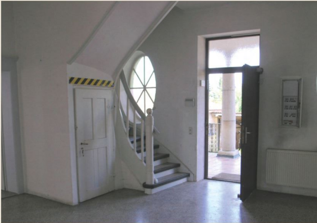
Ground floor foyer before renovation
